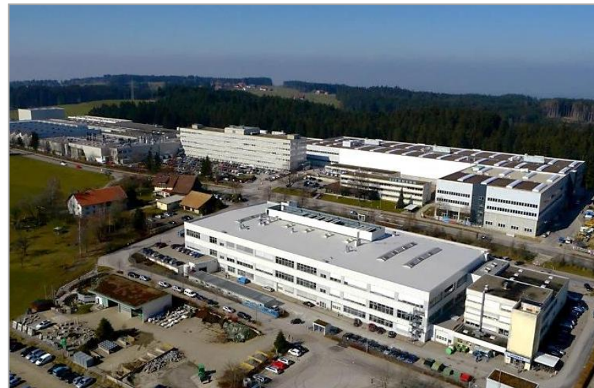
Liebherr-Aerospace site in Lindenberg
